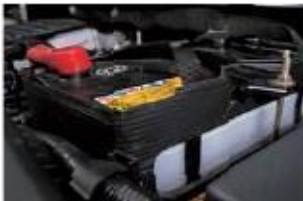
■ Battery Loose or corroded terminals
